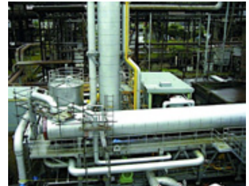
3.5 MW Kalina Cycle ® Energy Recovery Power Plant
